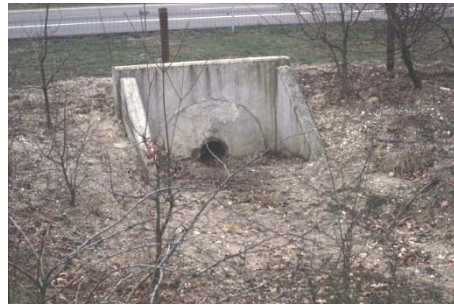
Figure.4 Badger tunnel realised in a road project (Photo Rob Jongman)
