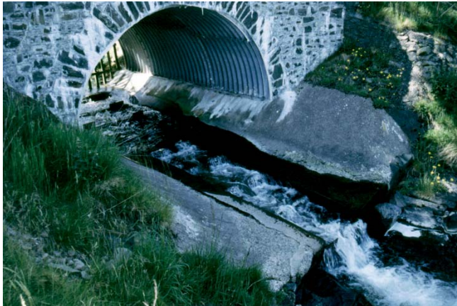
Figure 2: Fish ladder in one of the headwaters of the Tweed (Scotland) for migration of Salmon (Photo Rob Jongman)
