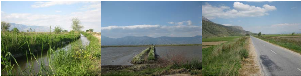
Figure 4: Infrastructure corridors, an irrigation canal (left); a drainage canal (center) and a road corridor (right)
